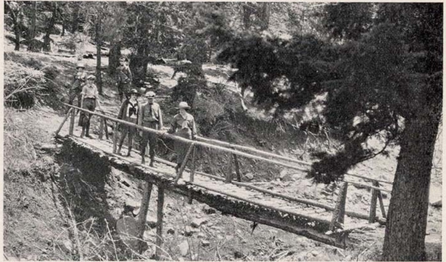
The Foot Bridge in Bear Gulch, a Short Distance Below Hosa Lodge, Genesee Park
